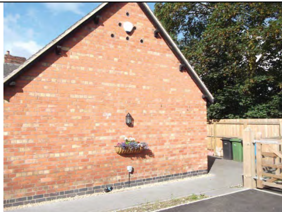
Holes for birds/bats into wall/roof cavity – east elevation
