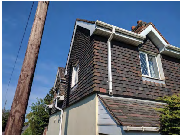
North and west elevations – tile hung
