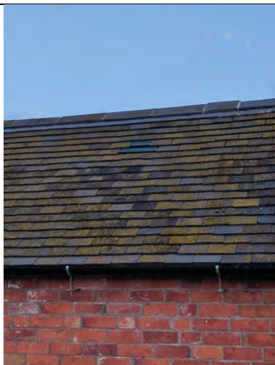
Bat access tiles in roof
