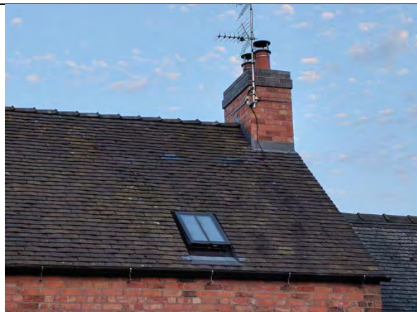
Bat access tiles in roof
