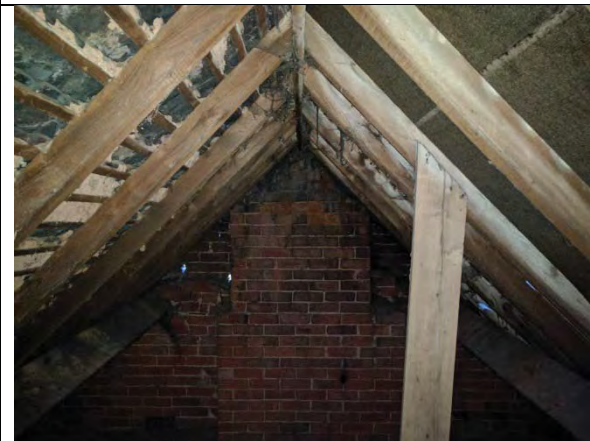
7. Typical roof structure
