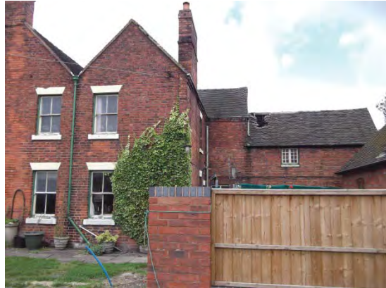
Farmhouse rear (south) elevation
