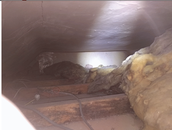
Northern roof void
