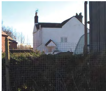
Rear (north) and side (east) elevations
