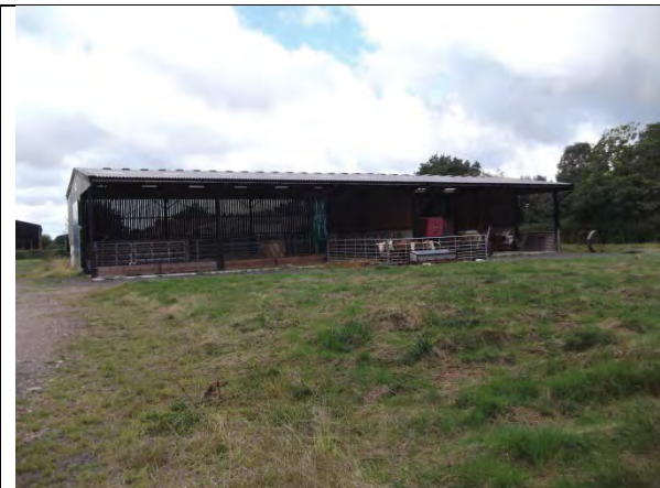
5. Barn – Negligible potential
