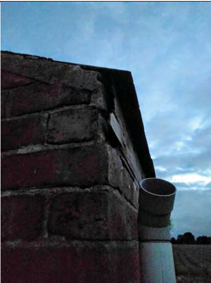
Building 1 – Timber Fascia
