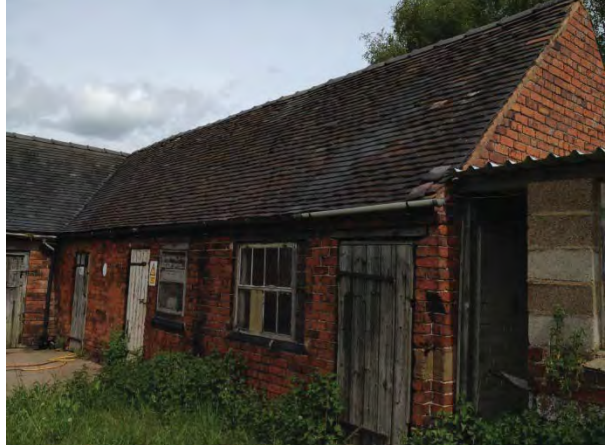
Front west elevation – chemical store.
