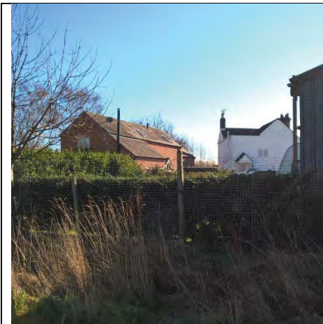
Front (west) and side (north) elevations
