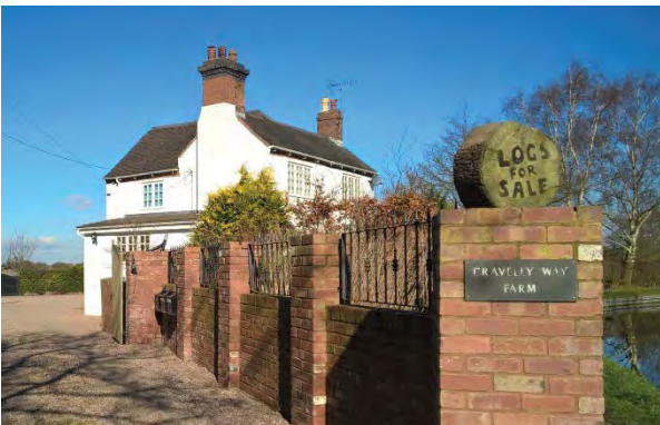
Front (south) and side (west) elevations
