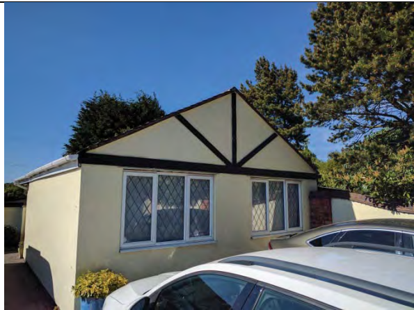
Converted garage – games room
