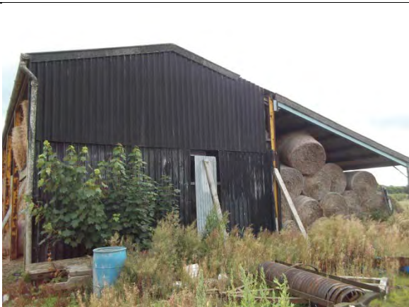
3. Barn - Negligible potential
