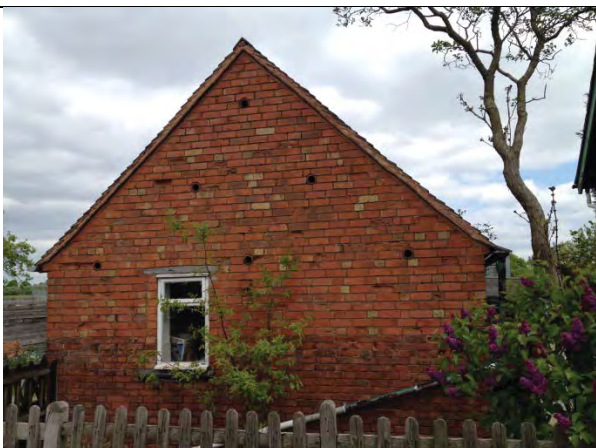
Outbuilding west elevation to road. Circular airbricks.
