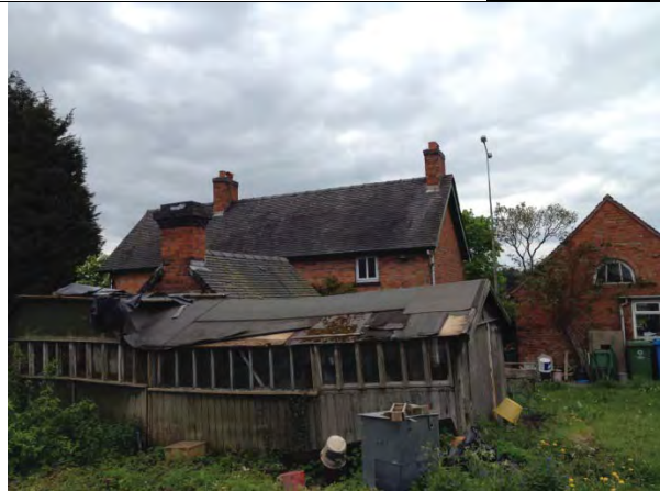
Rear (east) elevation and outbuildings.
