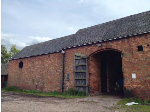
Rear (north) elevation with portal and barn doors
