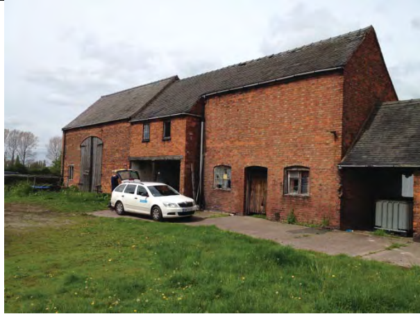
Front (south) elevation with open fronted areas.
