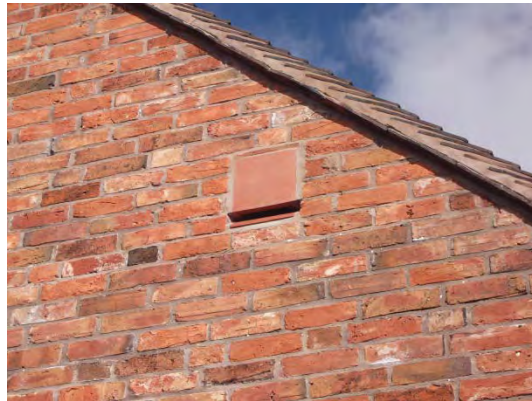
Rear (south) elevation showing bat box
