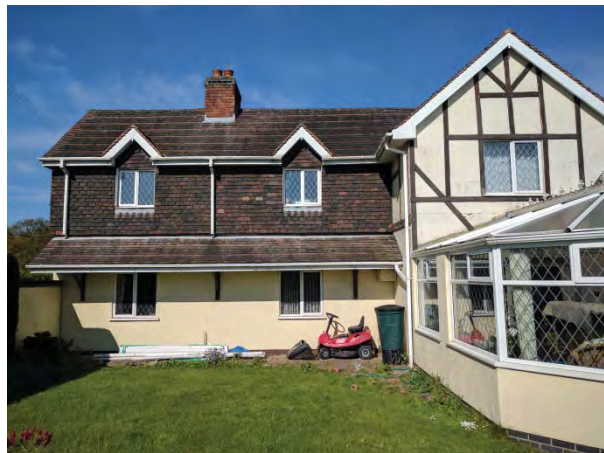
West elevation – tile hung
