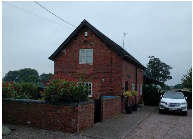
Front (east) and side (south) elevations
