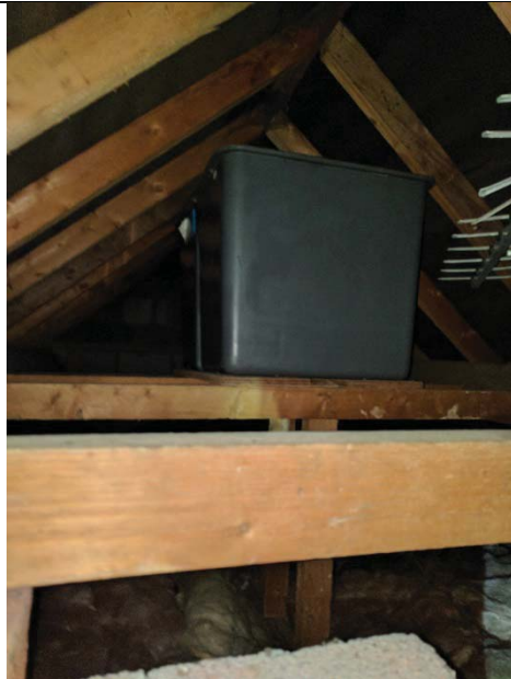
Southern roof void
