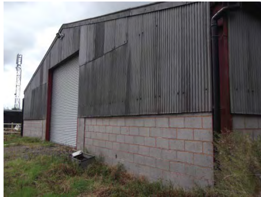
2. Barn – Negligible potential
