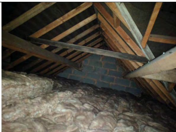
Southern roof void
